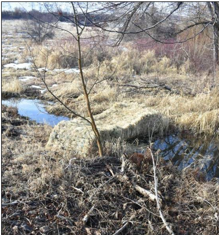
Hay bale put into overflow channel to reduce amount of water going over the road
