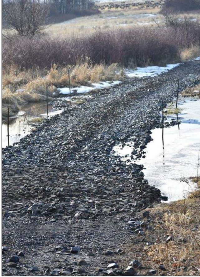
Additional rock on feed road
