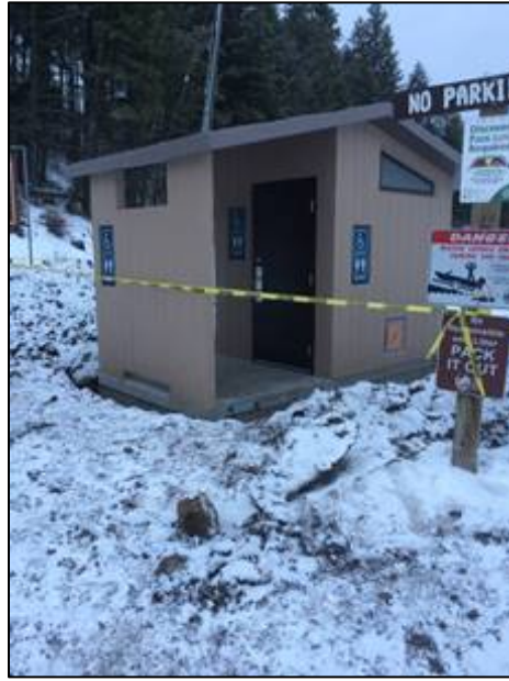
New vault toilet at Loon Lake
