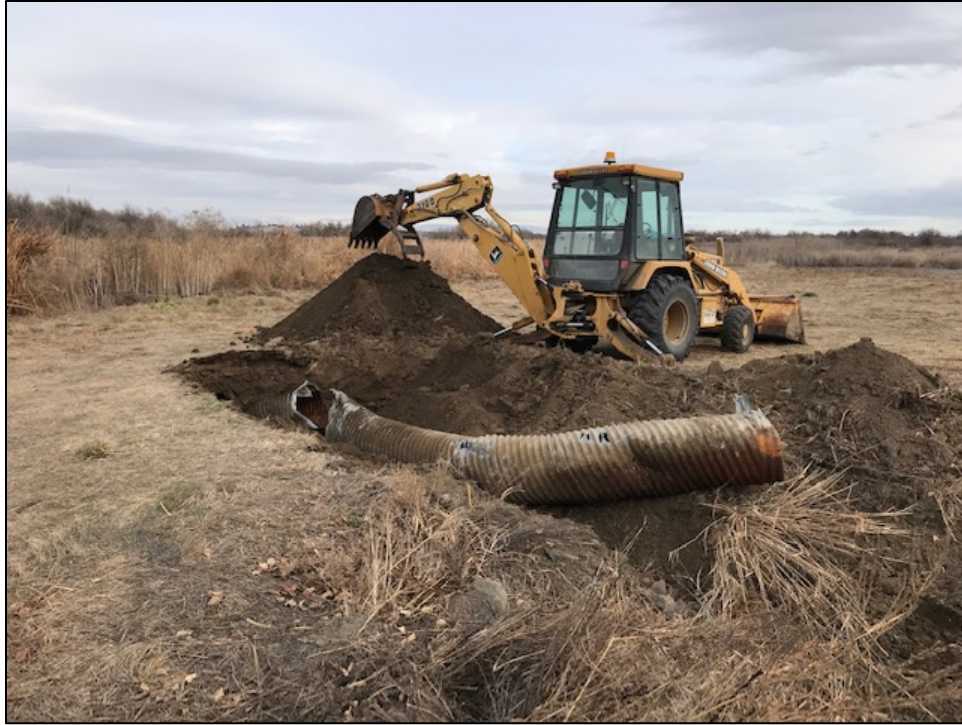
Old culvert about halfway removed
