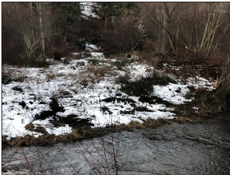
Area where machinery was in the water and clearing trees
