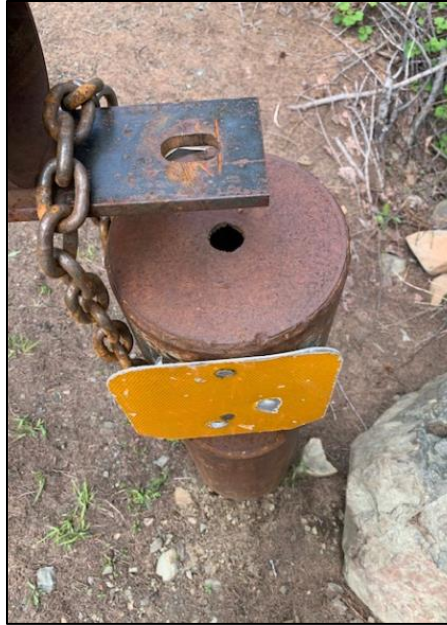
One of several gates that had their locks cut
