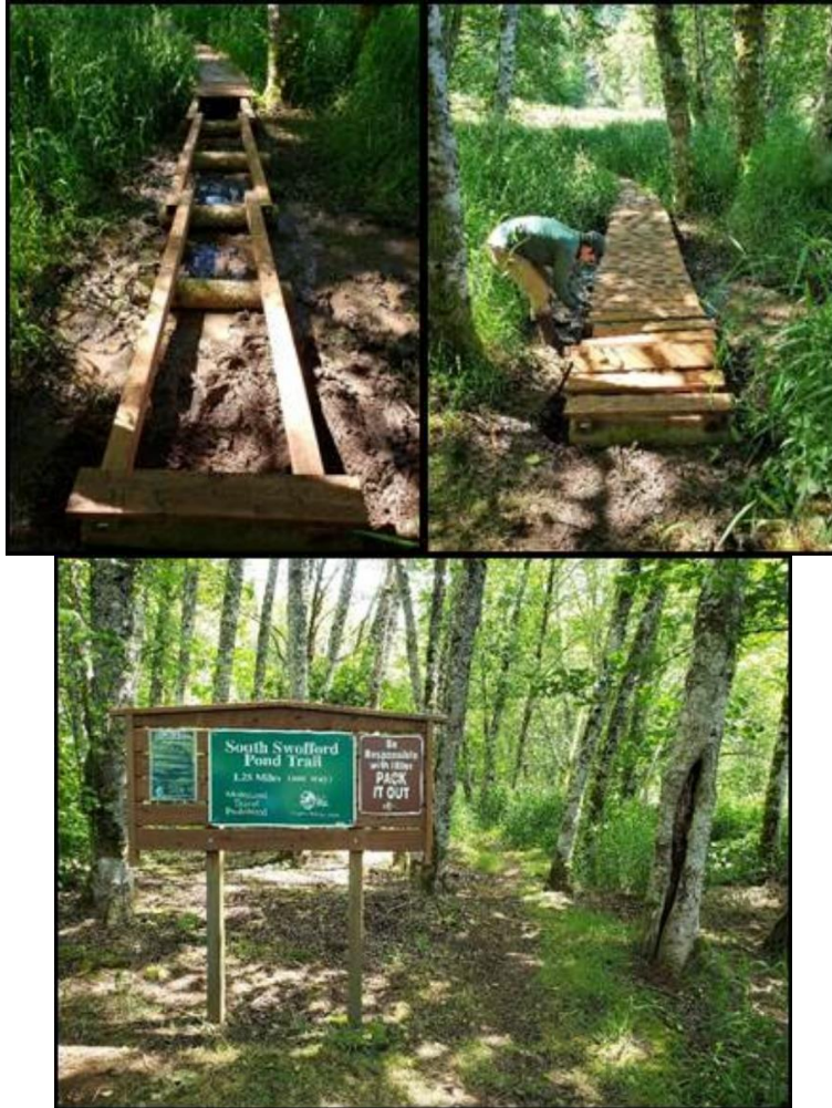
Swifford Pond Trail footbridge extension and a new kiosk
