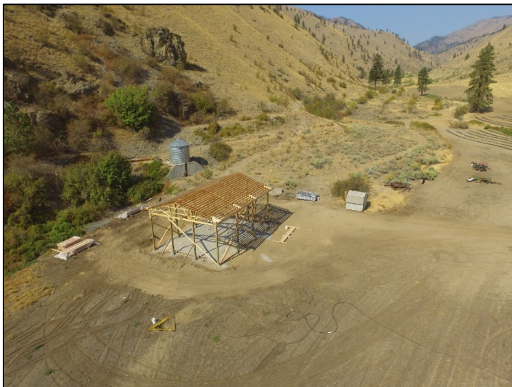
Swakane Storage and Shop Building – Photos by Daniel Hammerstrom, Glacier Industries
