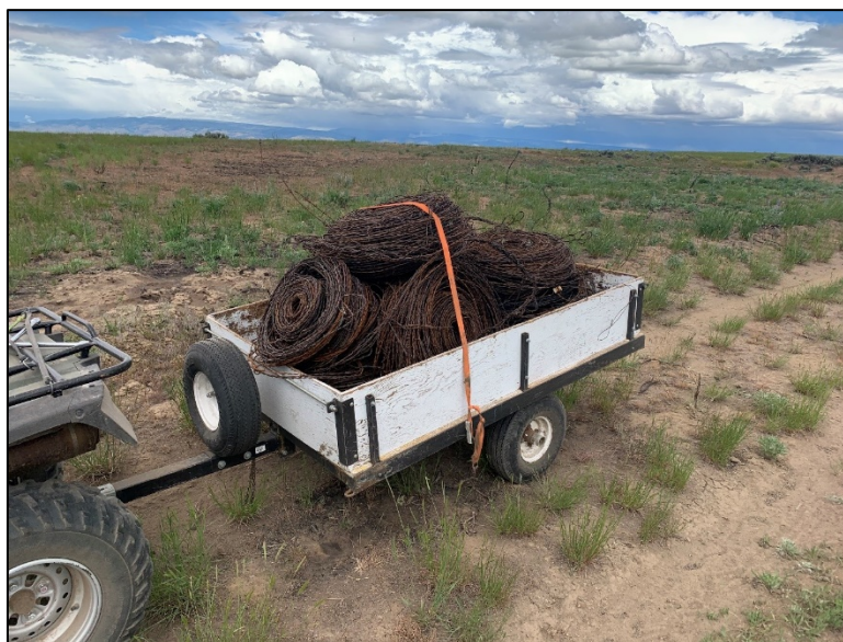
Barb wire rolled with machine roller and hauled off site
