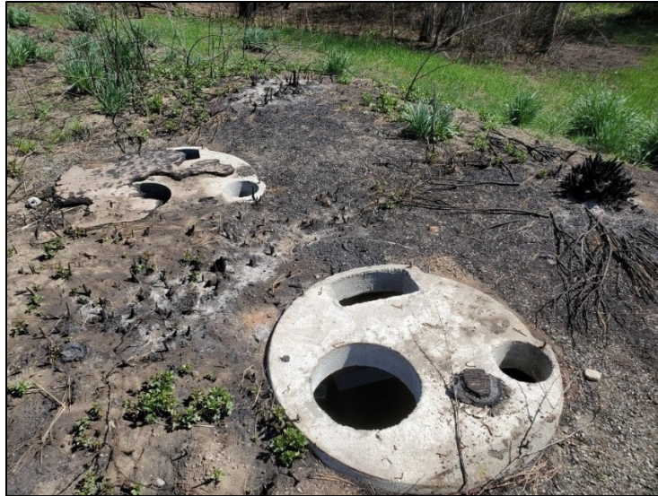
Latrine holes exposed by the Evan’s Canyon Fire
