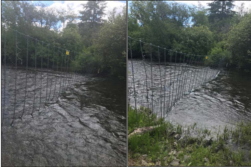
Taneum Fence in winter condition to pass flows (L) and Taneum Fence with summer elk panels to prevent elk from crossing (R)
