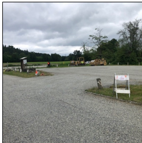
Crescent Lake South parking lots get a make-over in May 2021
