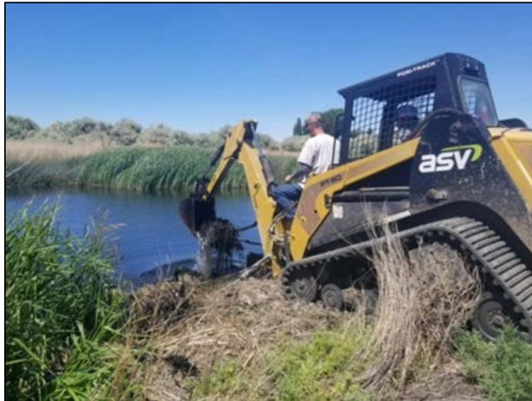
Water control structure being cleared of debris
