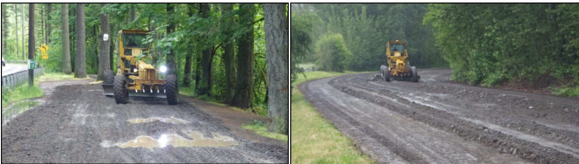
Grading at Barbers Access and Vancouver Lake
