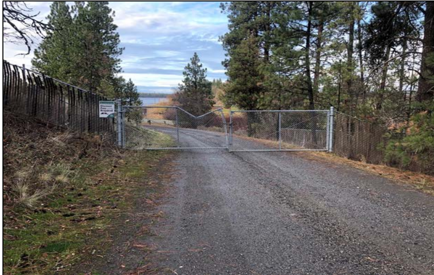
Clear Lake Water Access Area Locked Gate (bent frame is old damage)
