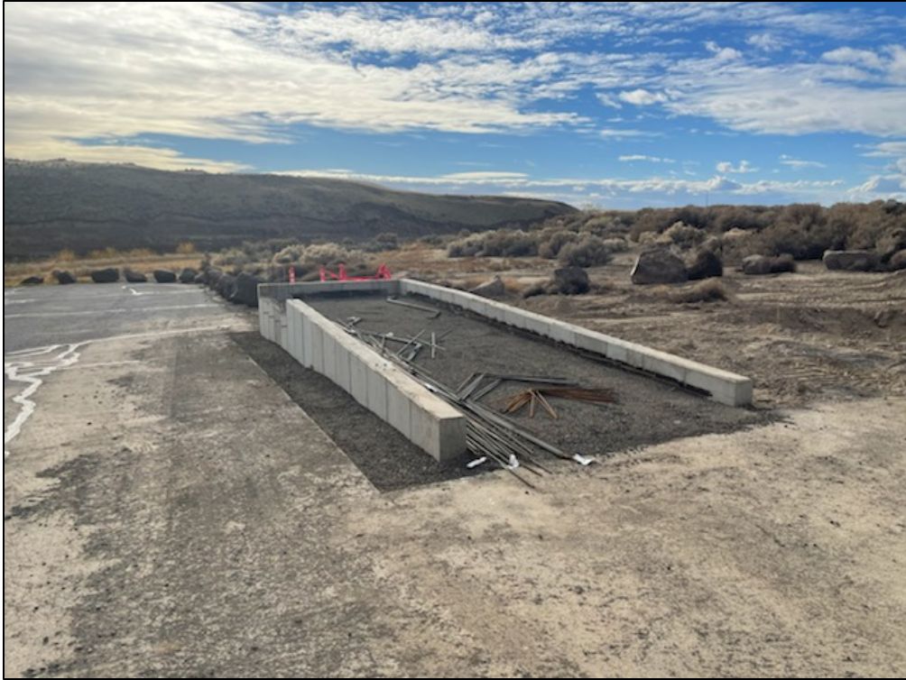
ADA loading platform in progress – Photo by Harmon
