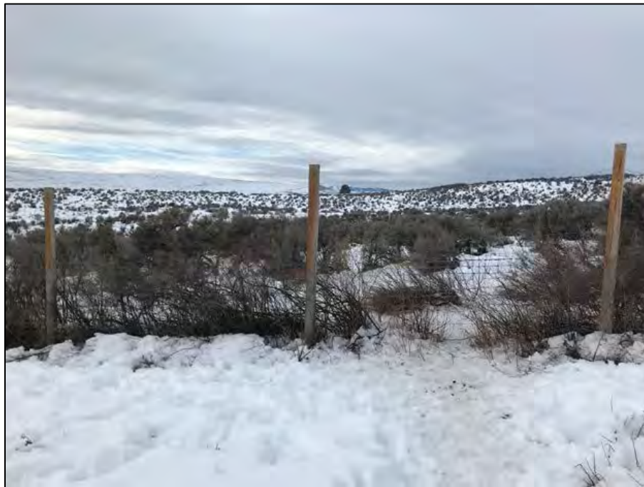
Damaged elk fence near Sunset Road
