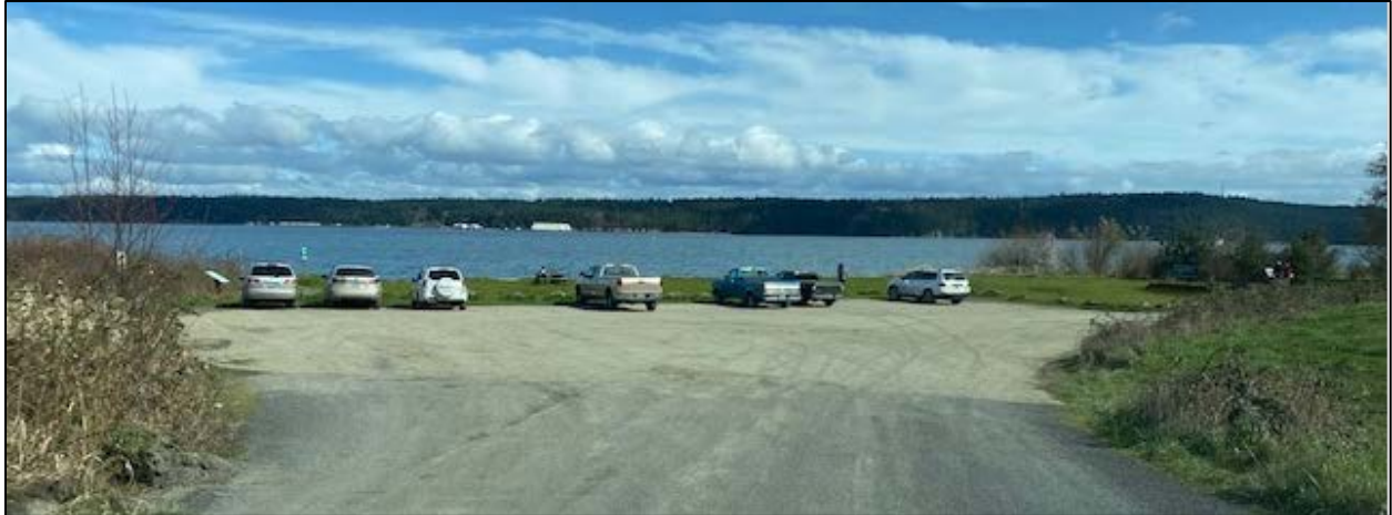
Irondale Access after repairs
