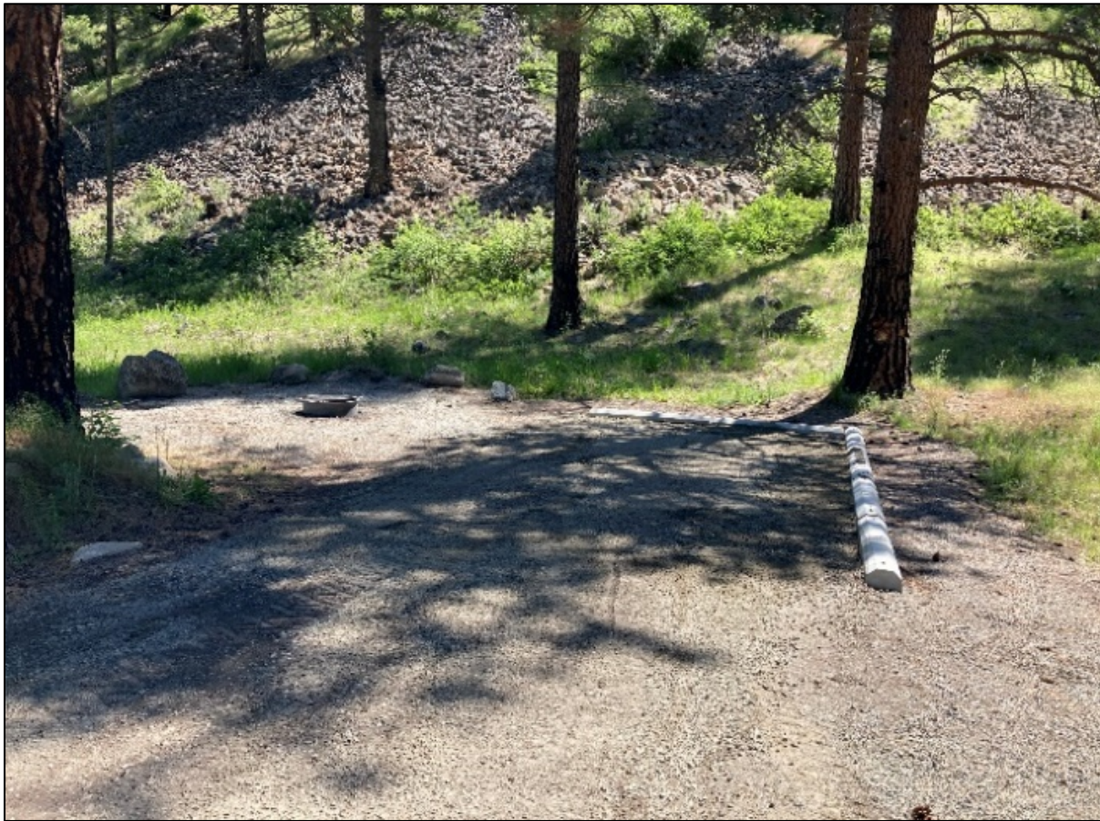
Finished camping pad with packed gravel, bumpers, and fire ring — Photo by N. Wehmeyer.
