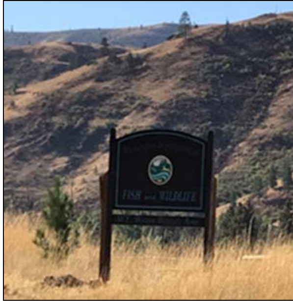
WT Wooten Wildlife Area entry sign was repaired and reinstalled
