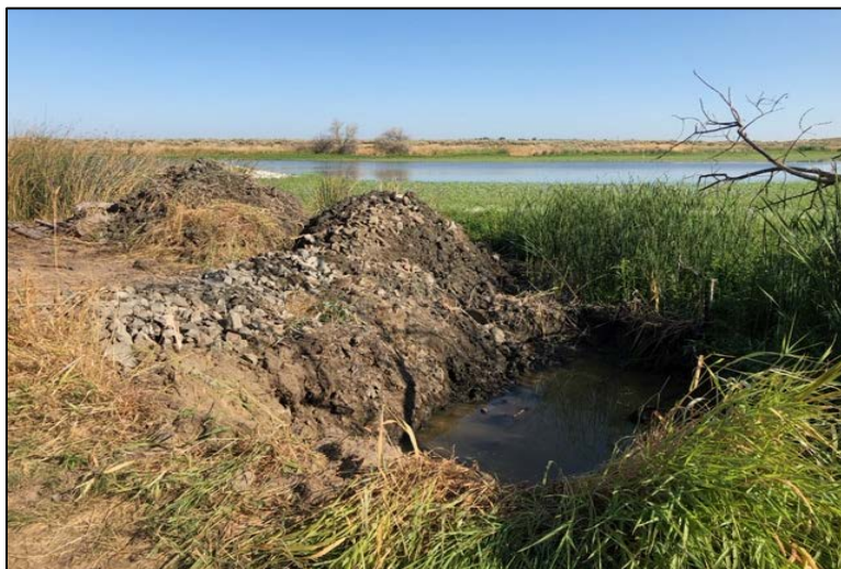
Site for new control structure
