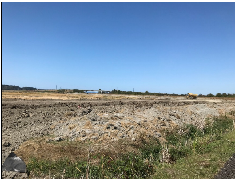
The beginning of the 0.7mile long berm that connects to the bridge in the background and will support an elevated trail
