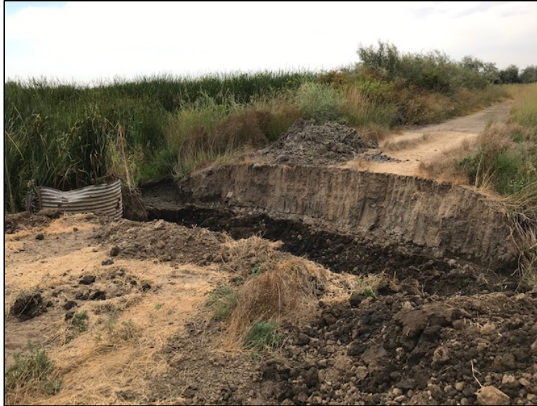
Site prepped for removal of old Giffin Lake water control structure
