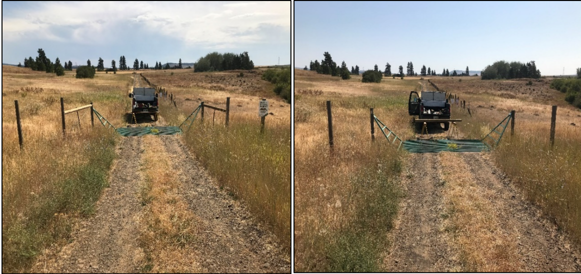
Horizontal brace post install, Hatchery Unit Before After
