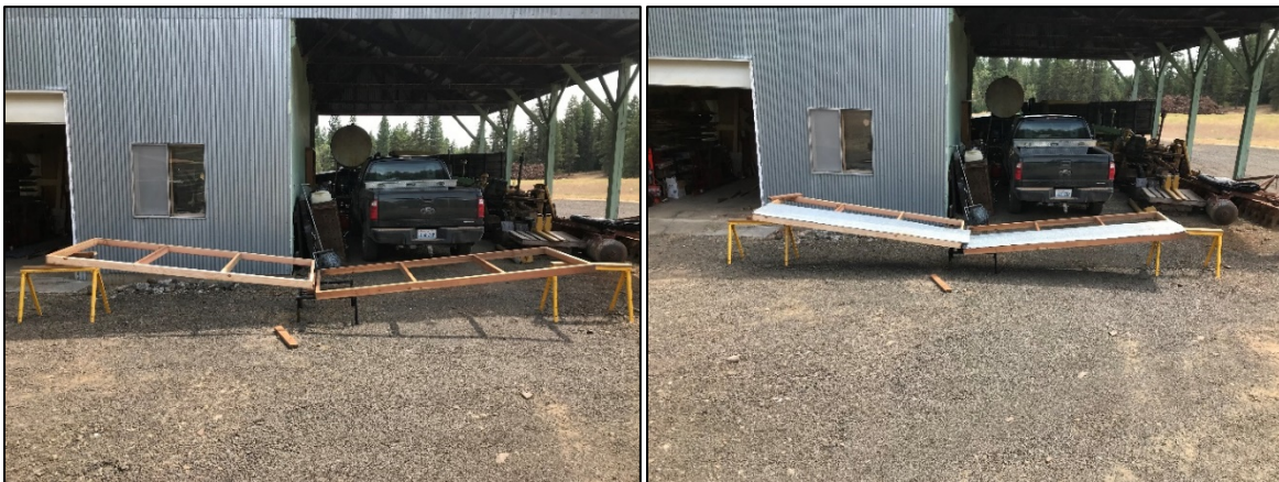
New rain catchment structures to be installed over wildlife guzzler
