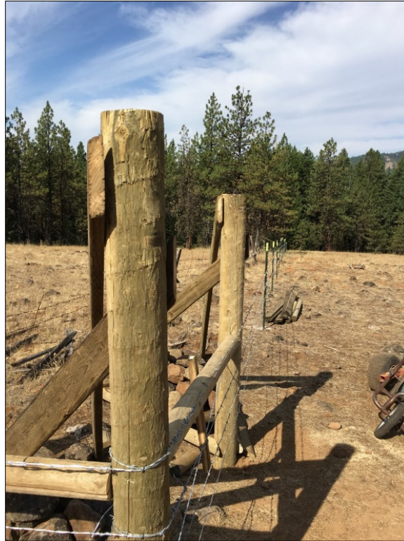
New corner brace built on the west side of the 4-O Ranch Wildlife Area
