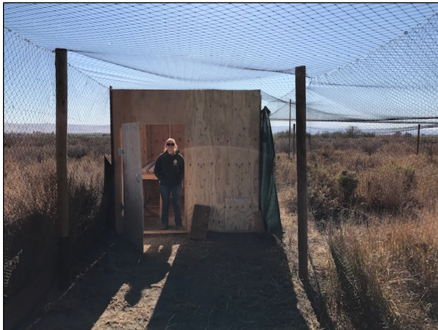
Front of pheasant catch chute. Small door on bottom right lets pheasants in. (Still needs a roof)
