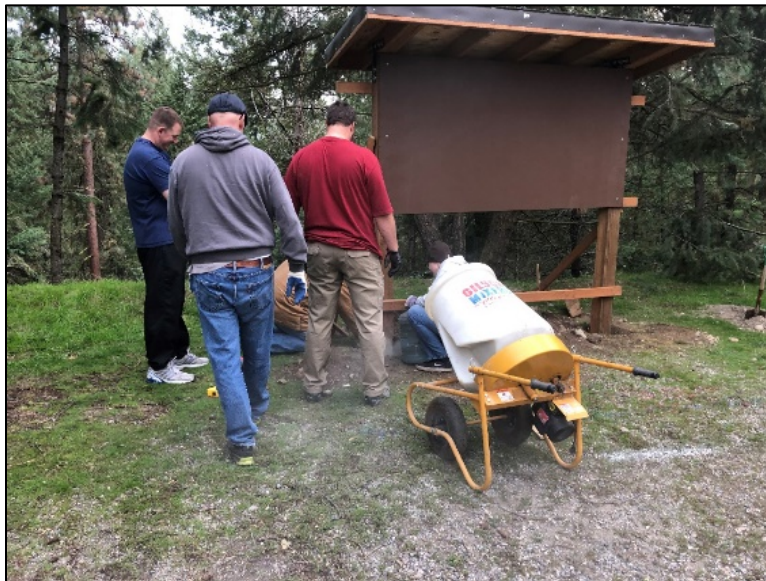
Pouring concrete for a secure footing
