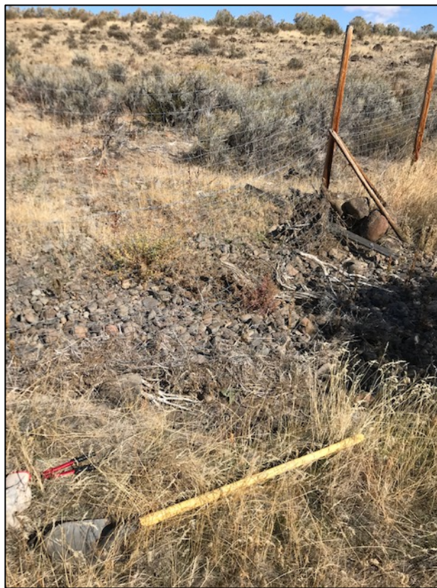
Hole in a breakaway area repaired
