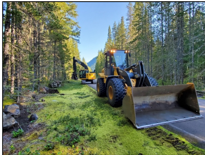
Merrill Lake boulder barrier installation
