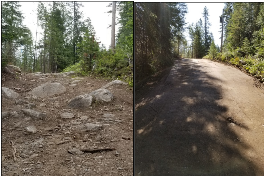
Caldwell Lake Access Road: Before (L) and After (R). Top gravel to be added at end of project work
