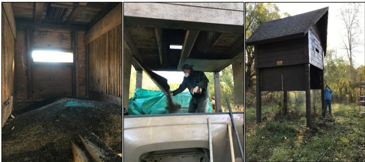
(Left) Guano piled up below the roosting baffles and flight training area inside the condo (Center) Biologist Atamian dropping the floorboards to empty guano from the bat condo (Right) INWC member Mike Curry power-washing the exterior of the condo
