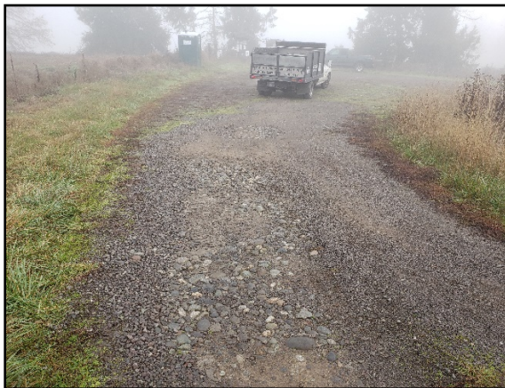
Pot hole areas along access drive into parking area also improved with gravel
