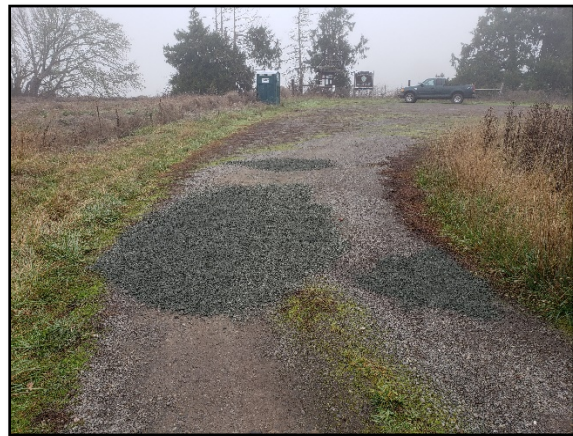
Pot hole areas along access drive into parking area also improved with gravel
