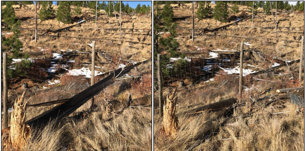
(Left) tree on elk fence and (right) repaired fence
