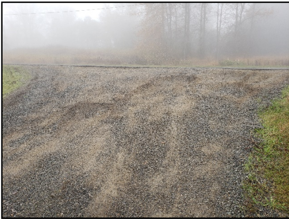
Access road into Lower Dungeness improved with gravel
