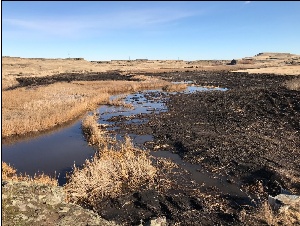
Revere wetland in process of being restored, looking east from control structure. The dark brown areas all used to be covered in 5-10ft tall rush and cattails, similar to what is visible on the left side of the photo
