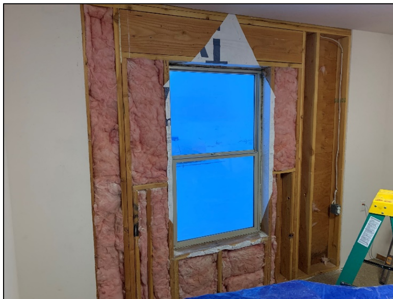
Swanson Lakes Wildlife Area Headquarters: Finch’s office ready for new window
