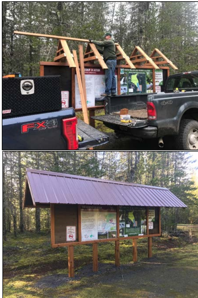
Under construction and finished photos of the Merrill Lake reader board
