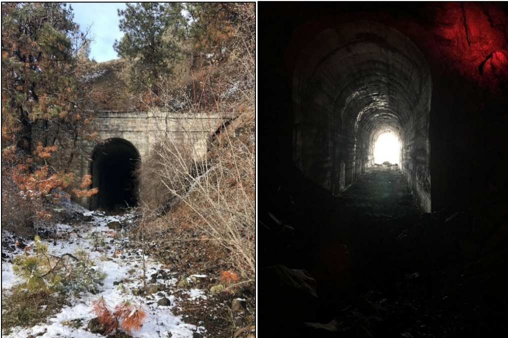
Abandoned railroad tunnel near Colfax investigated as potential bat hibernaculum
