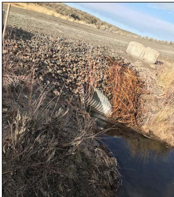
Herman Lake culvert post-cleanout, full flow – Photo by Jake Steele
