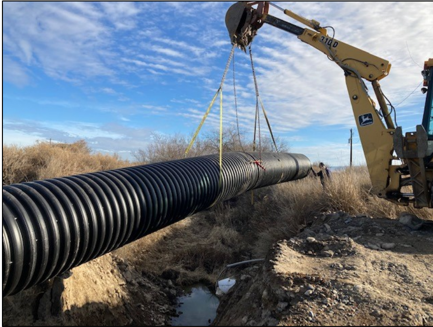
Lowering the new culvert pipe into position
