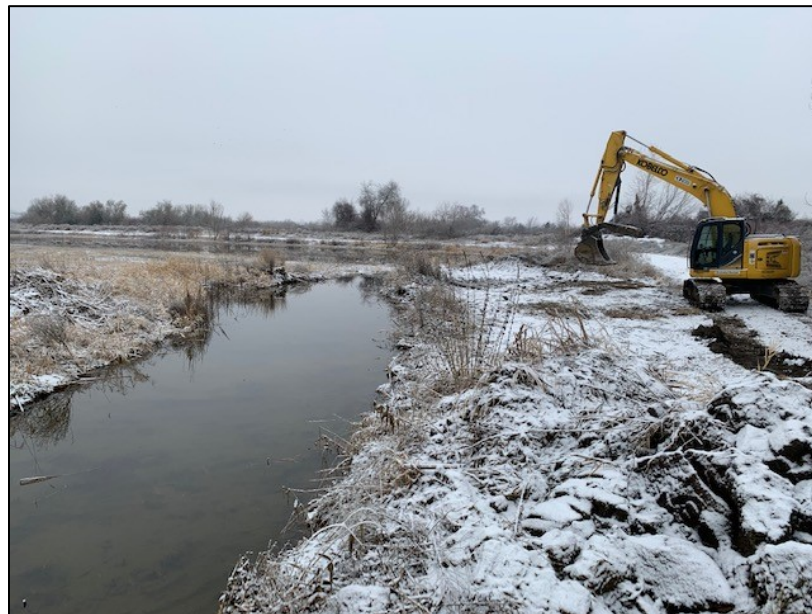
Johnson inlet ditch after widening and clearing debris
