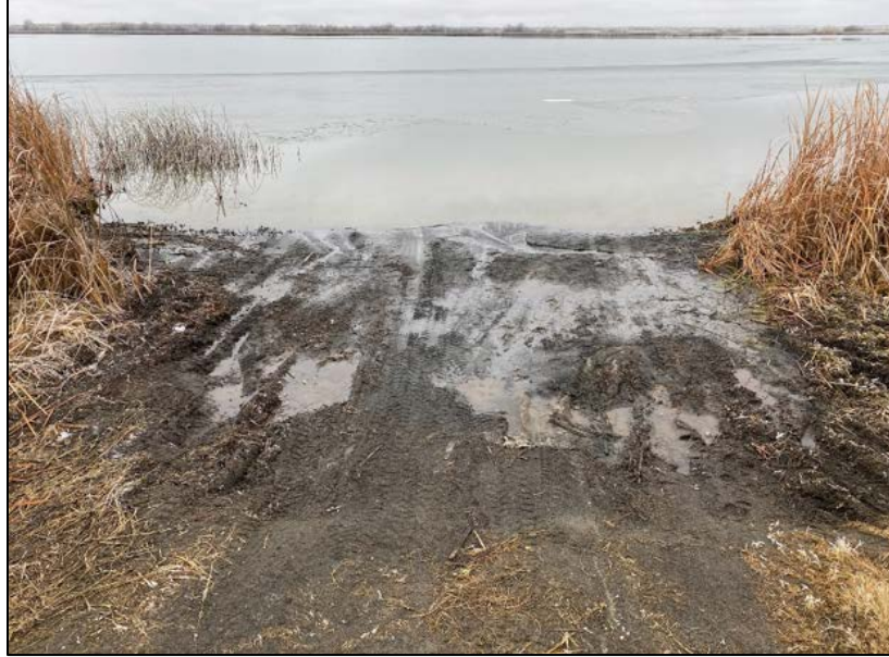
Road 2 northeast launch (before) – Photo by Manager Harmon
