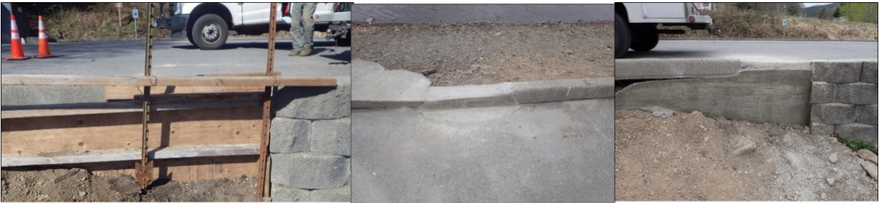
Repair of curb at Mineral Lake
