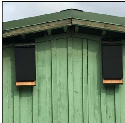
Maternity Bat Boxes Mounted on Shop in Onalaska
