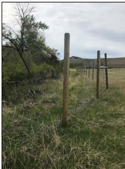
Break in perimeter fence utilized by elk at the Heart K
