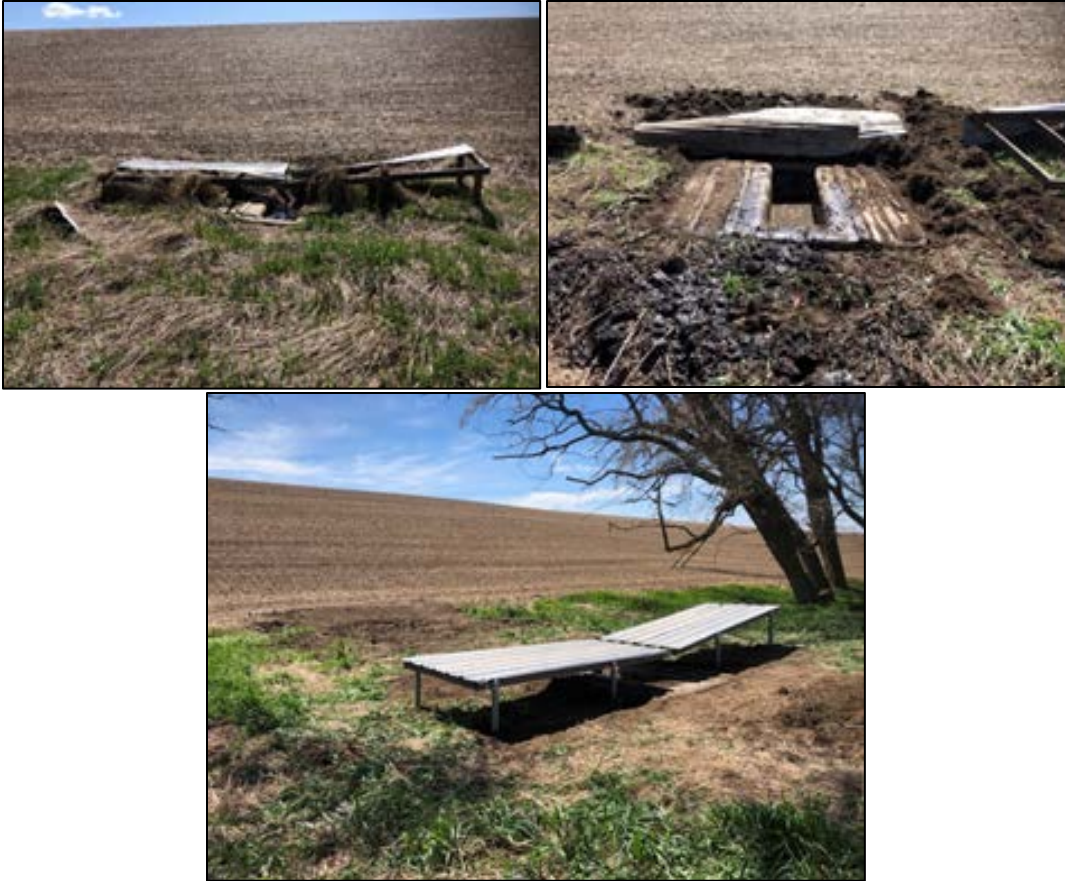
Wildlife Watering Facility guzzler removed and reinstalled. One of three guzzlers that were refurbished to working conditions on the WDFW access property
