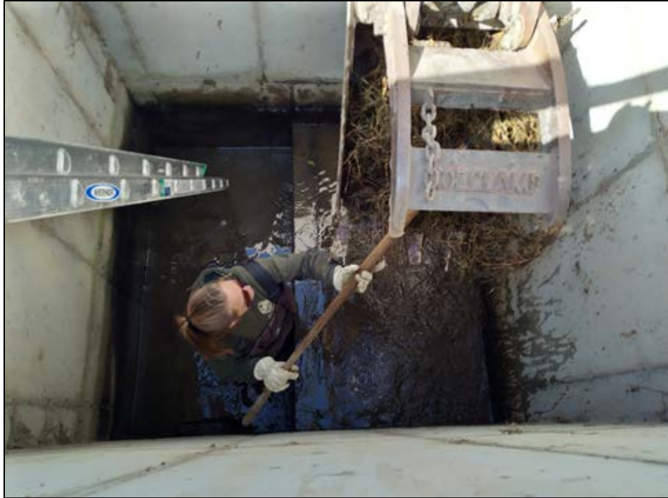
Natural Resource Technician Wascisin removing kochia “tumbleweeds” from Johnson Wetland weir box on Sulphur Creek
