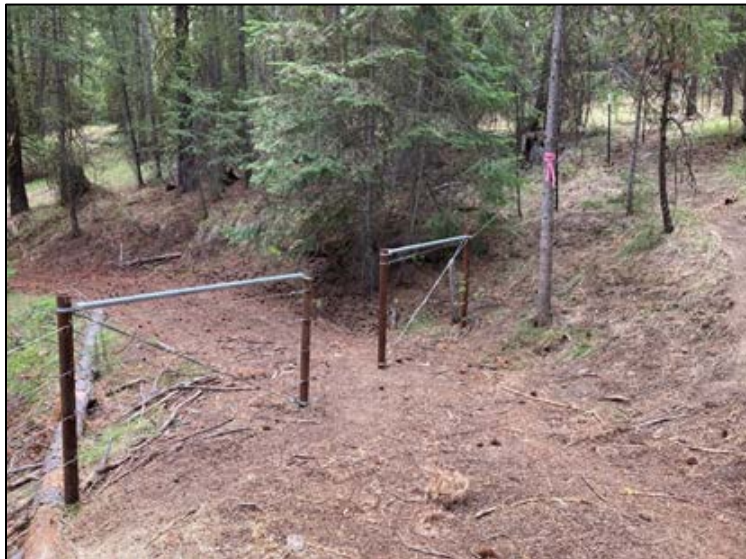
Walkthrough gate as part of the newly constructed fence at the Legoman Unit
