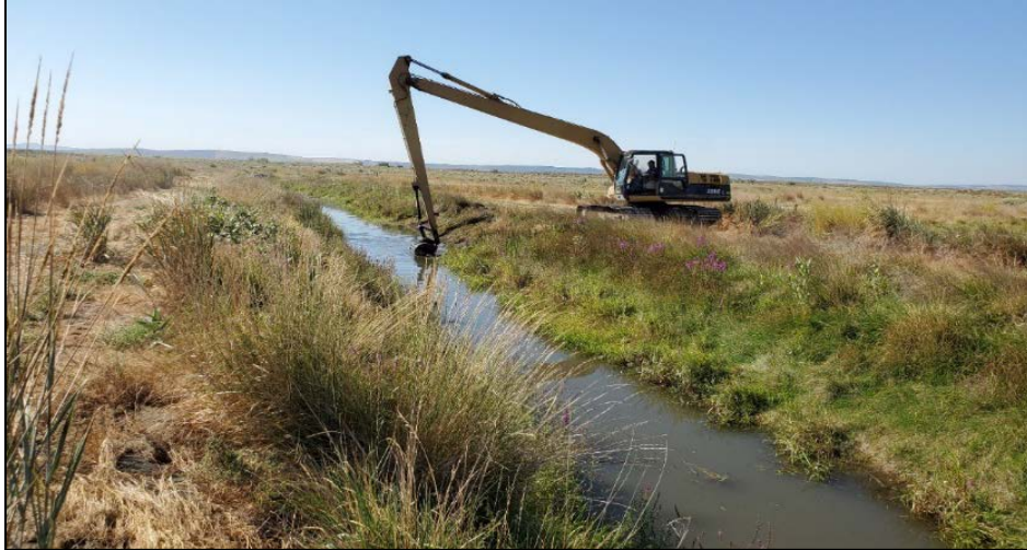
Delivery ditch cleanout at Winchester Regulated Access Areas – Photo by C. McPherson
