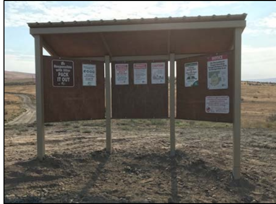
Replaced kiosk at Buffalo Parking Area
