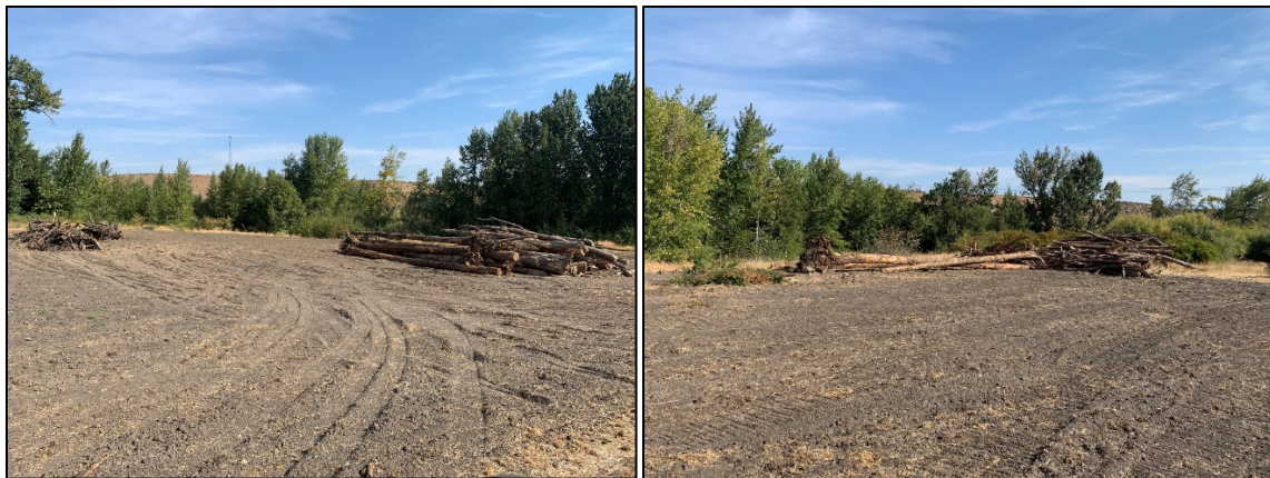
Material staged at the Ragheart site of the Taneum Creek Habitat Enhancement Project
