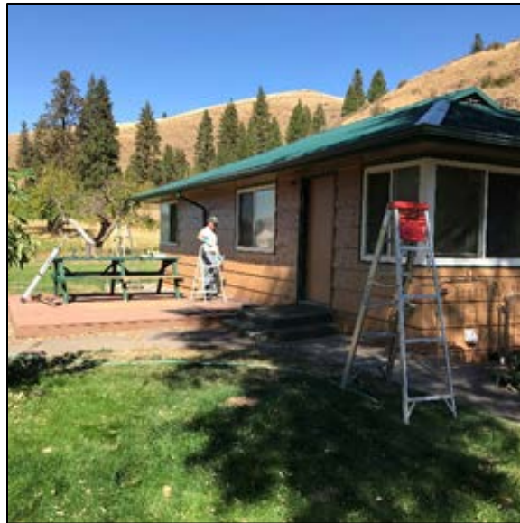
Natural Resources Worker Jensen caulking the windows after painting was completed
