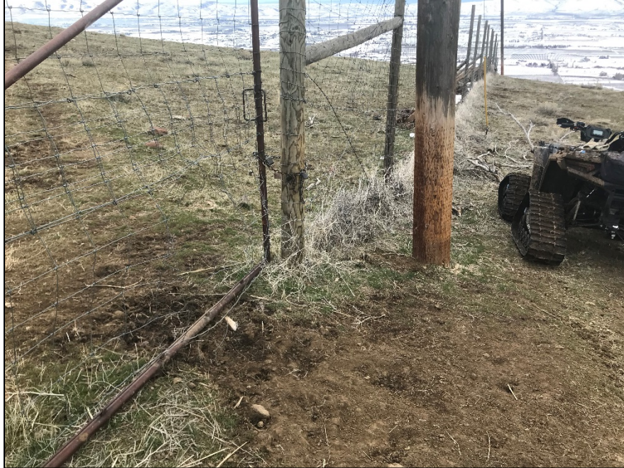
Hole in elk fence. Believe it or not, 36 elk went through this hole
