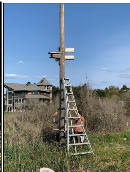
Installation of new boxes
