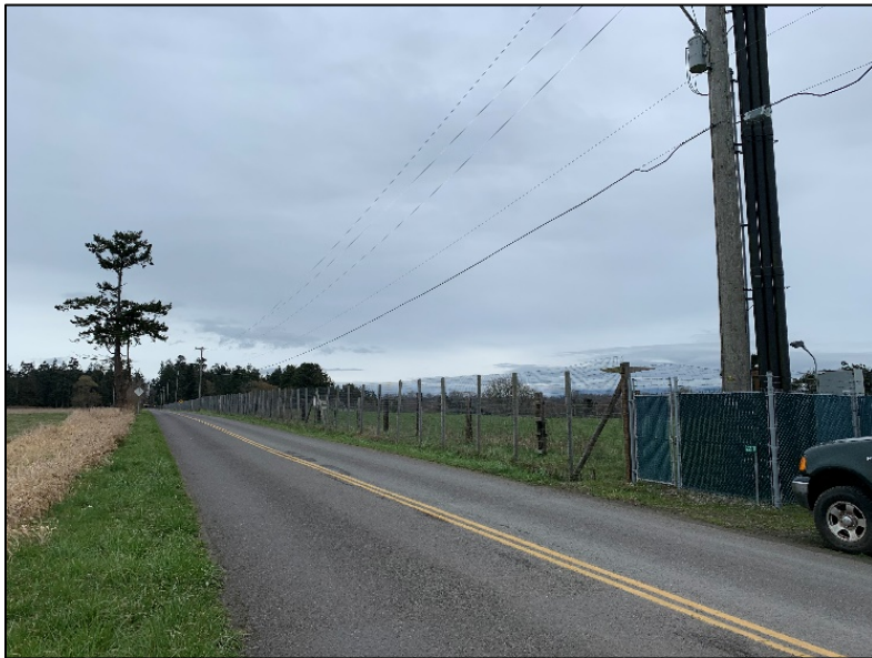
Power lines/pole near the Olympic Game Farm
