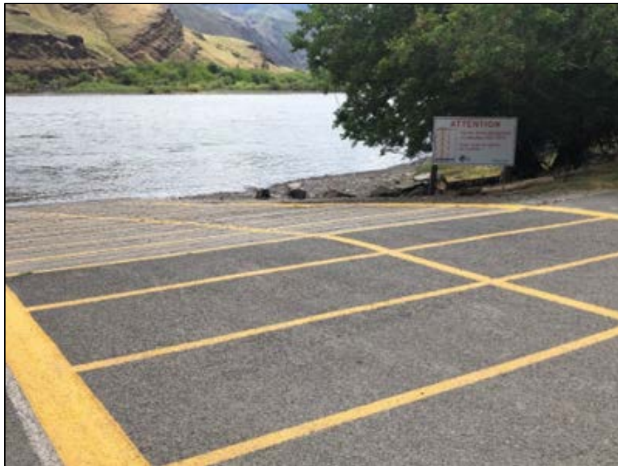
New striping and sign at Heller Bar Boat Ramp
