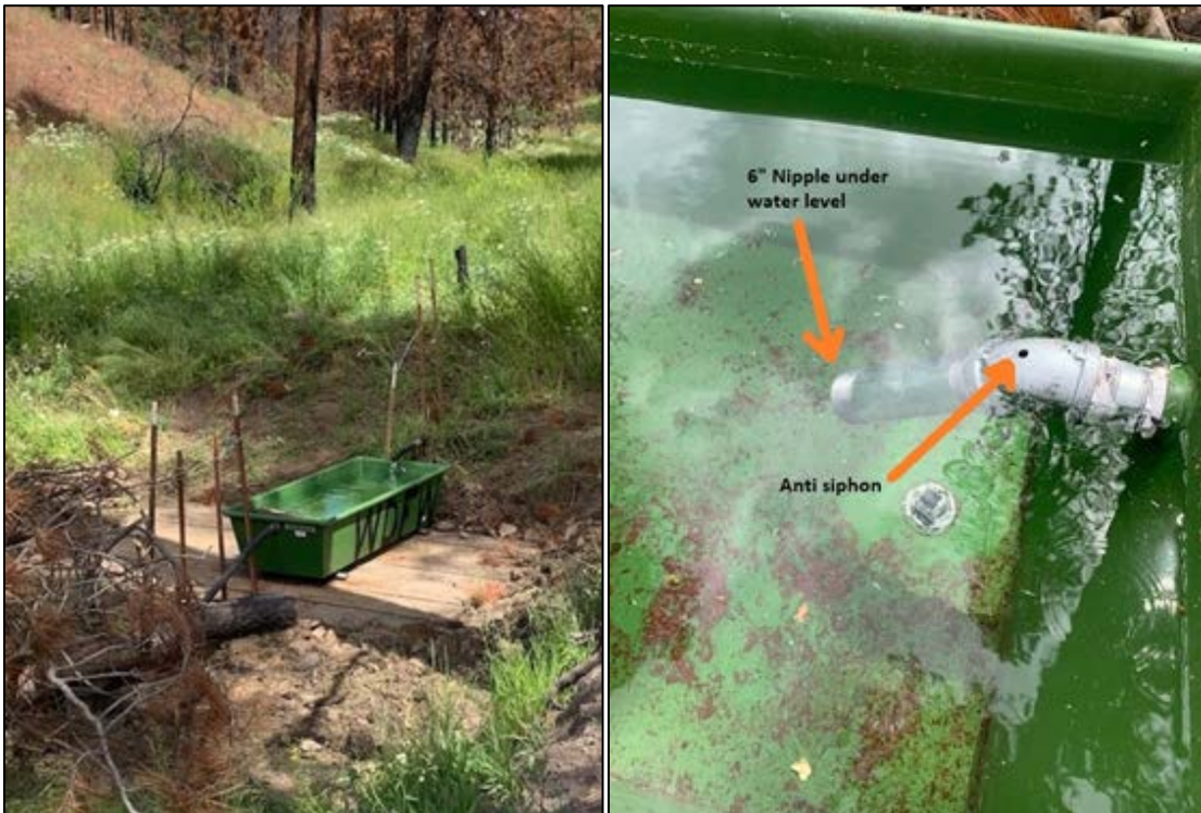
Newly Replaced water trough as a spring enhancement for wildlife and recreational users
