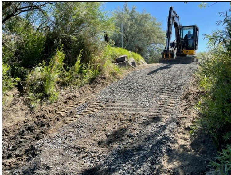
Hyde Street Access site after launch improvements
