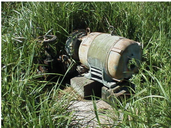
Photo 3 & 4. Unnamed pond and tributary to the Methow River. An illustration of the large 50 horsepower pump and small priming pump needed to irrigate the large plot of land WDFW manages. The intake at this site was considered to be adequately screened.
