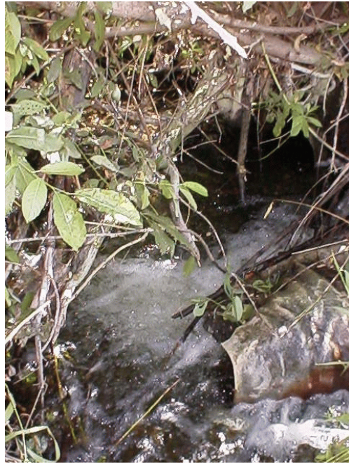
Photo 7. Alder Creek (48.0296). With the series of three culverts being installed at this crossing, it was inevitable that it would eventually become a fish passage barrier for resident salmonids.
