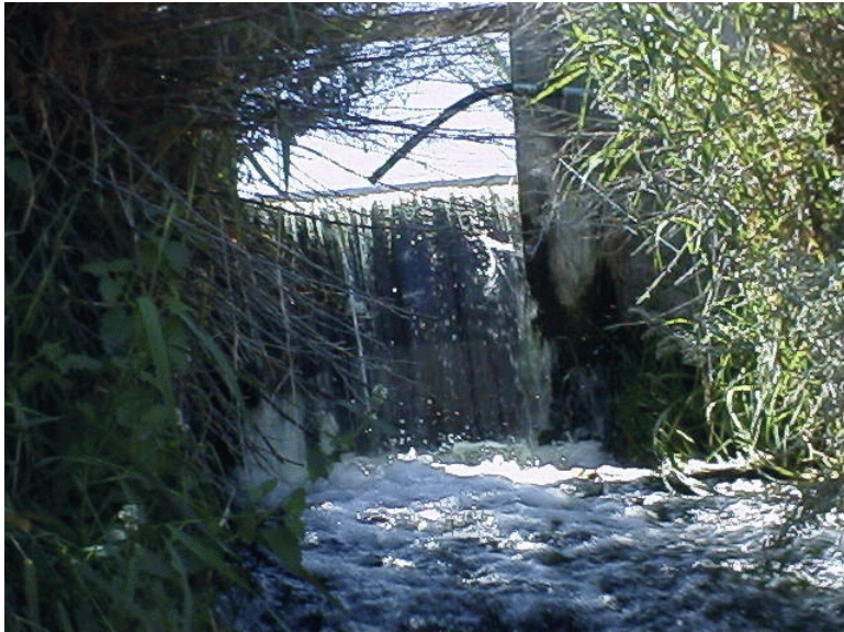
Photo 5. Chiliwist Creek (49.0034). The dam at the point of diversion was a total barrier to fish migration at the time of inventory and requires redesign to allow for 100% fish passage throughout the year.
