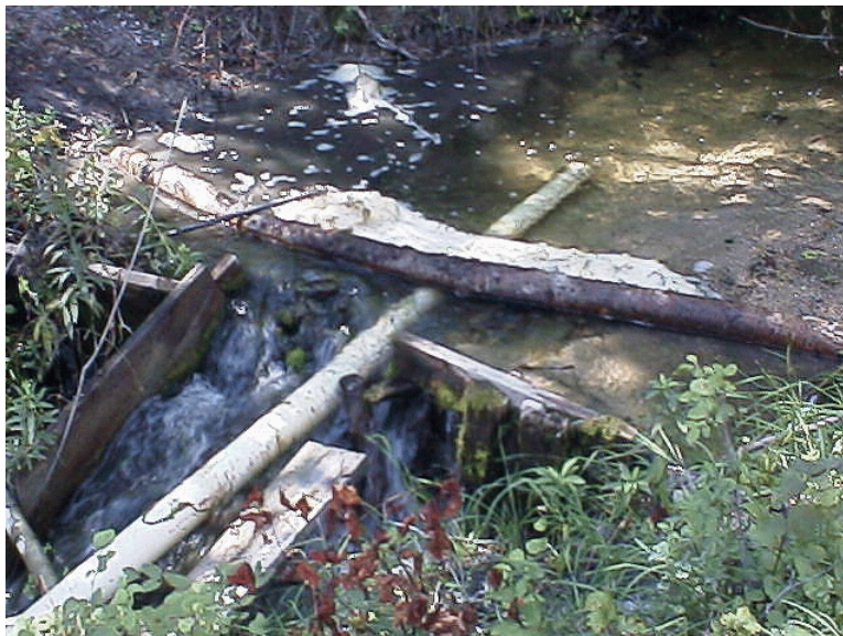
Photo 6. Alder Creek (48.0296). A perfect example of the various types of unscreened hydraulic diversions located within the Methow Valley. This diversion is utilized as an auxiliary water source to a much larger diversion from the Methow River. The 4 inch pvc pipe is diverting water into the larger canal downstream.
